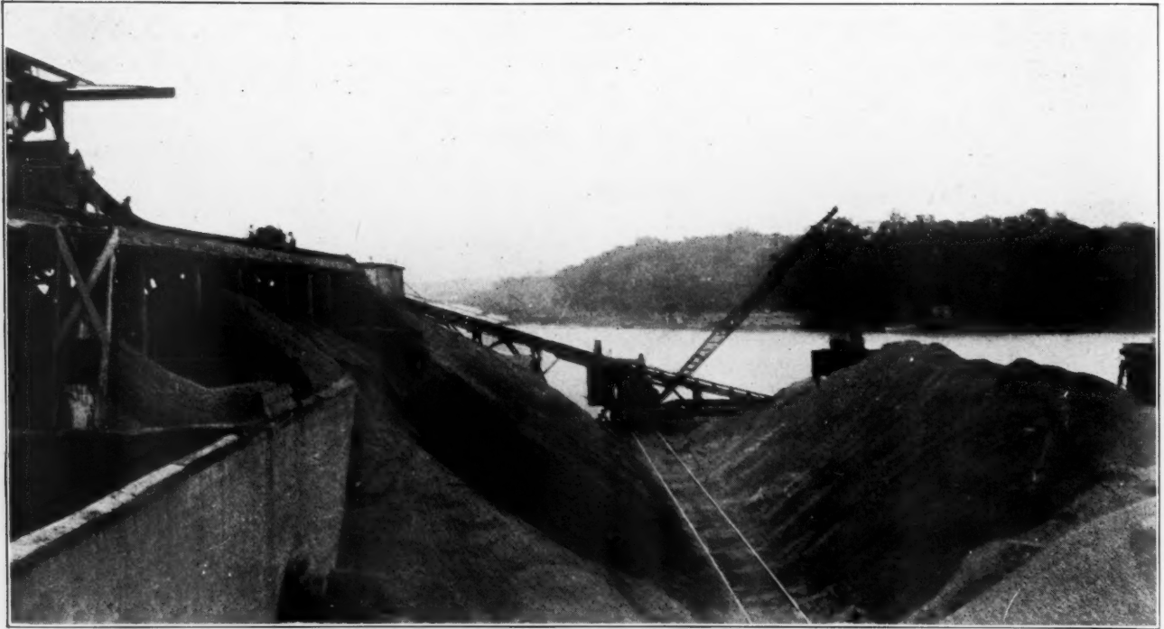
Stockpiling System, Excess Material Spills Over Concrete Bins and is Handled by Locomotive Crane
